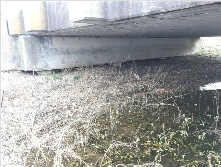
Abutment - Bent 3: Settlement of end-slope
