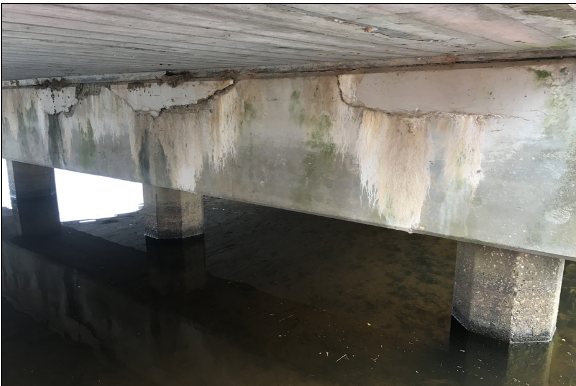
Cap - Bent 2 back right: Cracking/delamination
