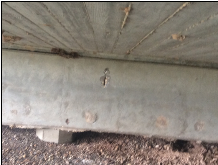
Abutment bent 3 spall with exposed rebar
