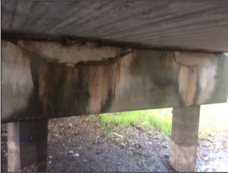
Bent 2 cap has spalls and Delams.
