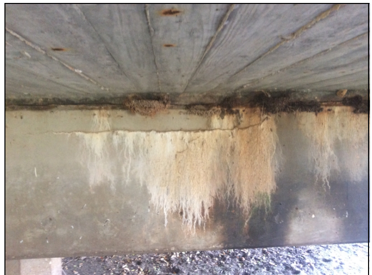
Cracks with with efflorescence on cap 2 behind
