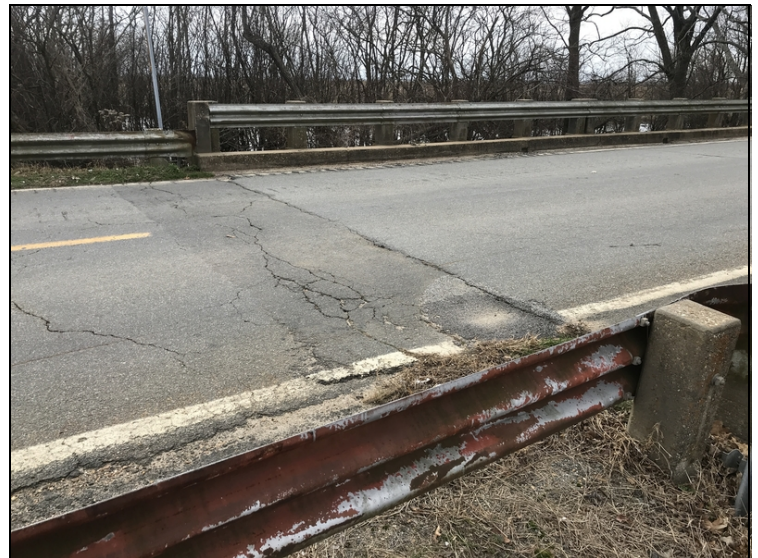
Approach roadway - Bent 3: Deterioration/settlement
